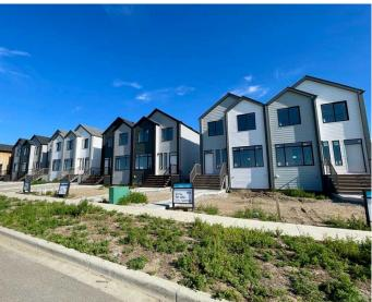
ConstructionVinyl Siding, Wood Frame, ConcreteFoundationPoured Concrete
